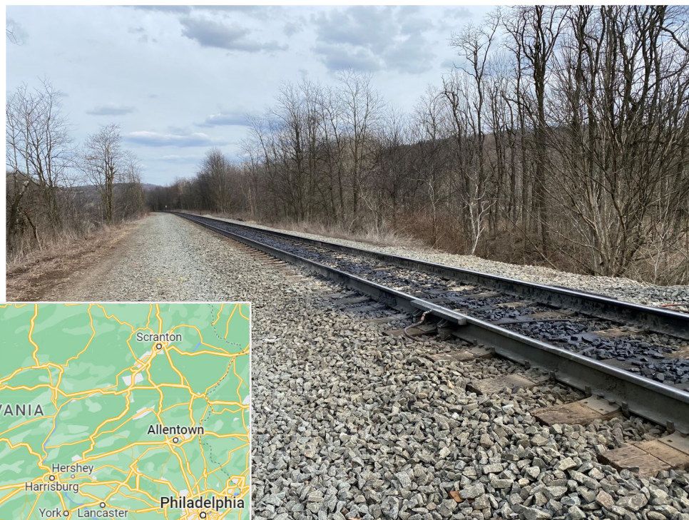
Tunnelhill (fouled ballast)
